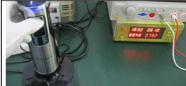
64. Low voltage start test
