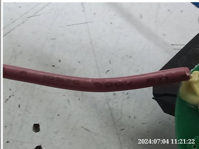
Photo# 65 Internal construction check
