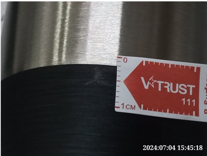
Photo# 12 Poor painting - minor
