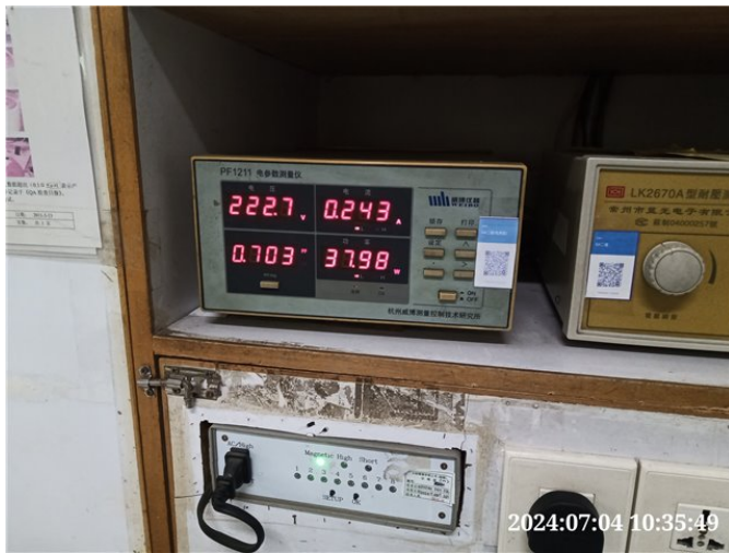
Photo# 95 Power consumption test(motor appliance)
