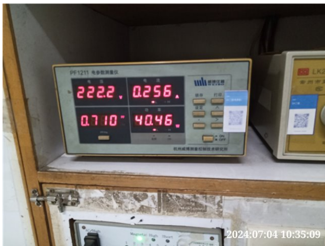
Photo# 93 Power consumption test(motor appliance)
