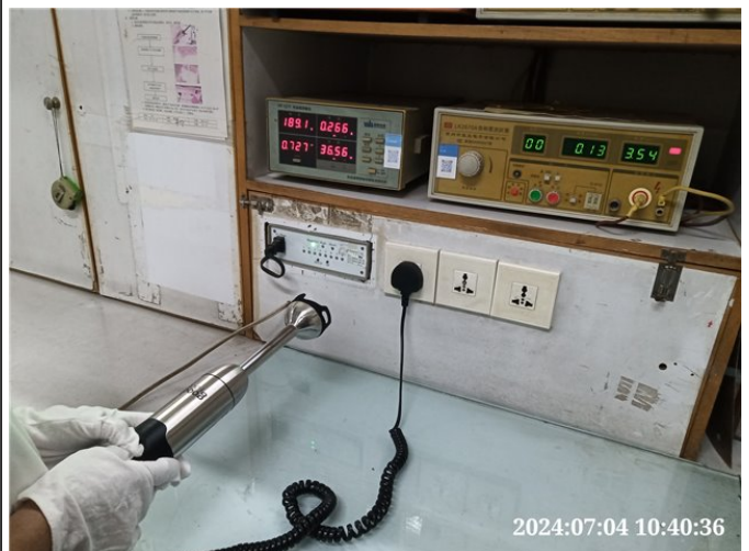
Photo# 26 Low voltage start up check
